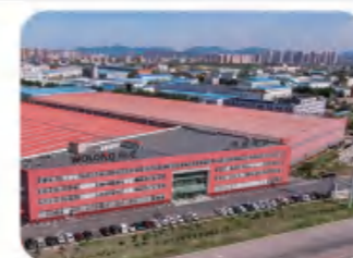
鞍山 | 驱动+新能源 Anshan - Driver control + New energy
